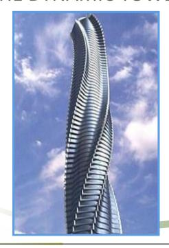
The wind turbines will be located between two consecutive floors, while the solar panels will be placed on top of each floor and the roof. The wind turbines will be capable of producing 1,200,000 kilowatt hour of energy, and both the energy sources combined can generate enough surplus electricity to power several nearby structures. An intelligent building as such that can power itself is environmental friendly to a huge extent.
