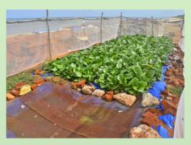
root-microorganism' contact made in these units, over 80 % of wastewater treatment is completed quickly (in about 2 hours) as compared to 2 days or more needed in other systems.
