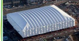
one of the largest ever built for temporary use. In terms of design, it's more of a tent or scaffold that's Next there's the **Water Polo Arena**, the first ever dedicated Water Polo venue built for the games. The 5,000 person capacity arena holds a 37-meter pool and a uniquely sloped roof (from 25m down
