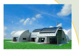
lar. The arches also collect rainwater which can be directed to above or below ground storage. Above ground storage would also be solar heated.
