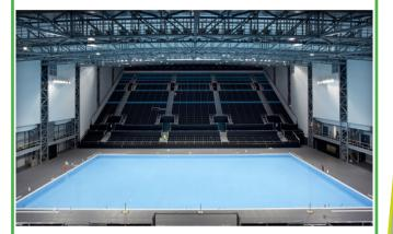
to 6m). But more interestingly, the arena was built sustainably such that it will be torn down immediately after the games, and the materials reused for construction. The building is made with Polyvinyl chloride material, or PVC, which is easily recyclable.
